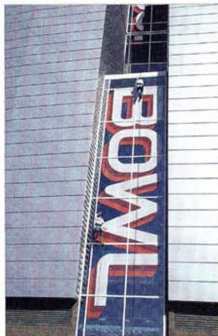
Roe employees installed this 75' window perf on the stadium by repelling.
